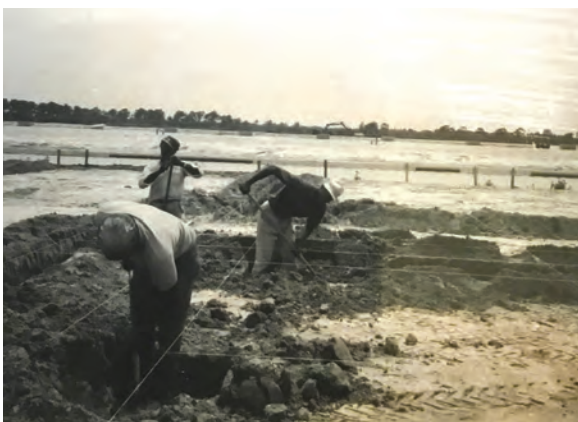
Digging the footers
